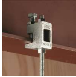
Universal beam clamp for standard beams
